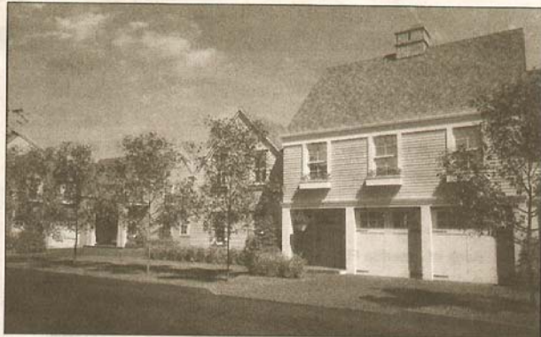
Palmer Hill, located at 77 Havemeyer Lane in Stamford, is a luxury condominium and townhomes community being built by development team Buckingham Partners and Sun Homes.
